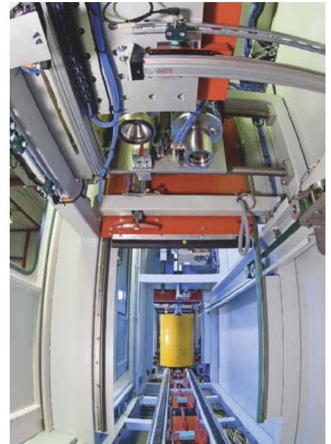
The conveyor technology allows a process which is both safe and fast
