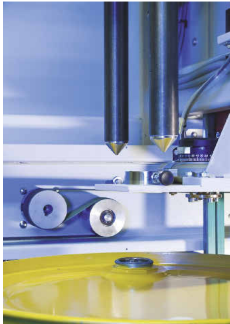
Future-proof filling plant due to modernisation of safety standards
